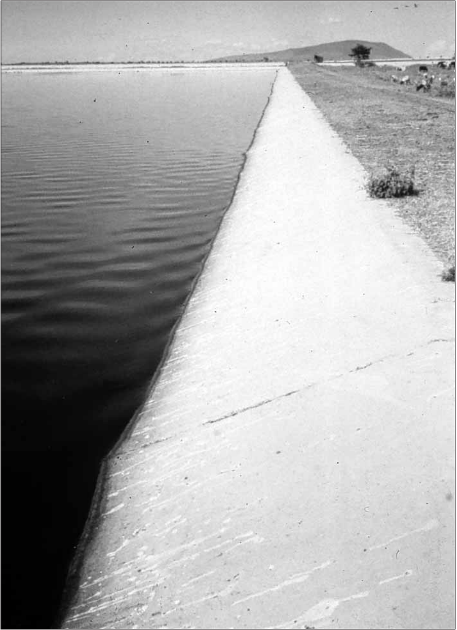
Figure 13.1 Embankment Protection by Concrete Cast in situ
