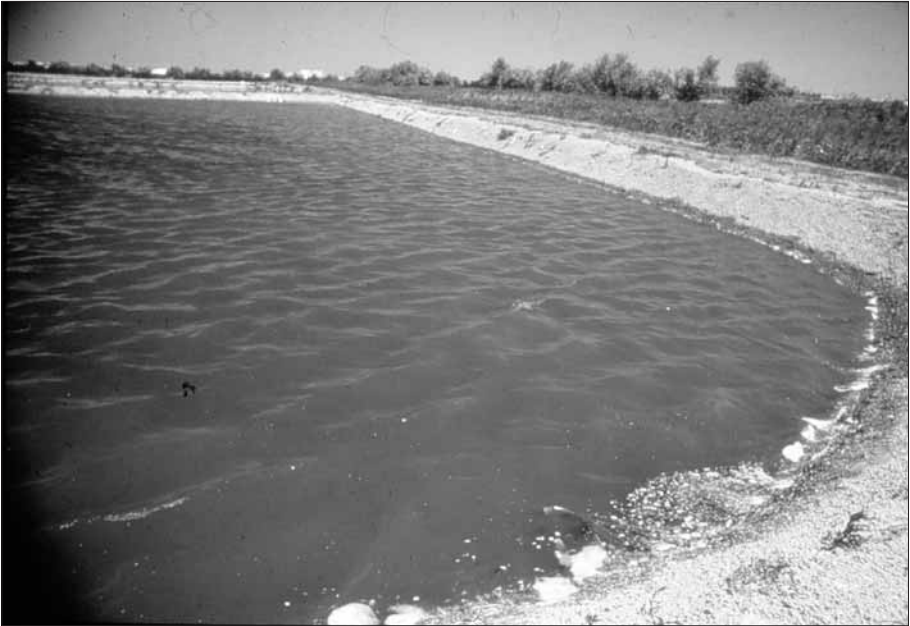
Figure 13.3 Embankment Protection by Stone Rip-rap
