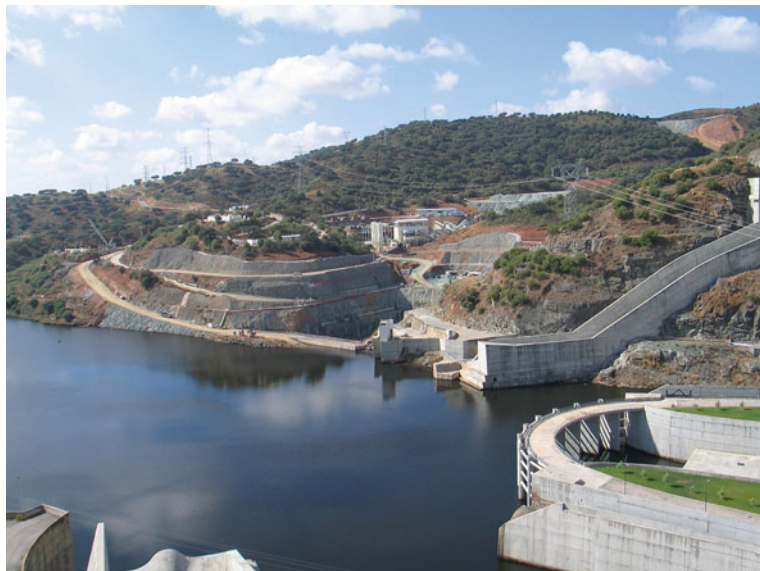
Fig. 12.2 Guadiana dam, Portugal
