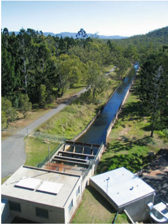
Fig. 12.5 Irrigation channel, North Queensland
