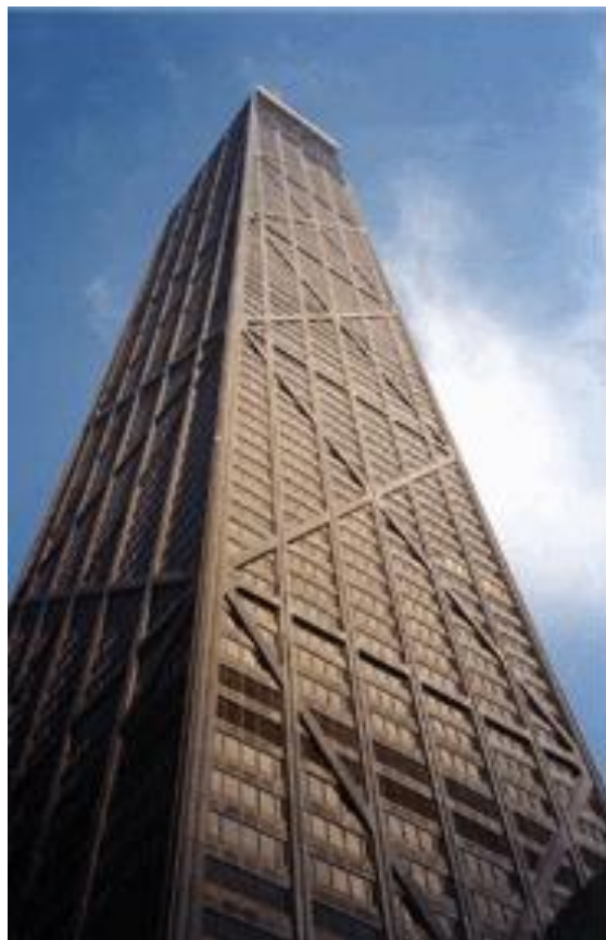
Figure 14.4 – Hancock Center, Chicago
