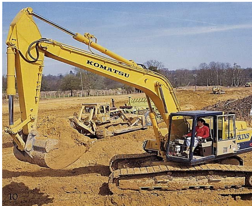
Figure 8.4 – Excavator digs and moves earth
