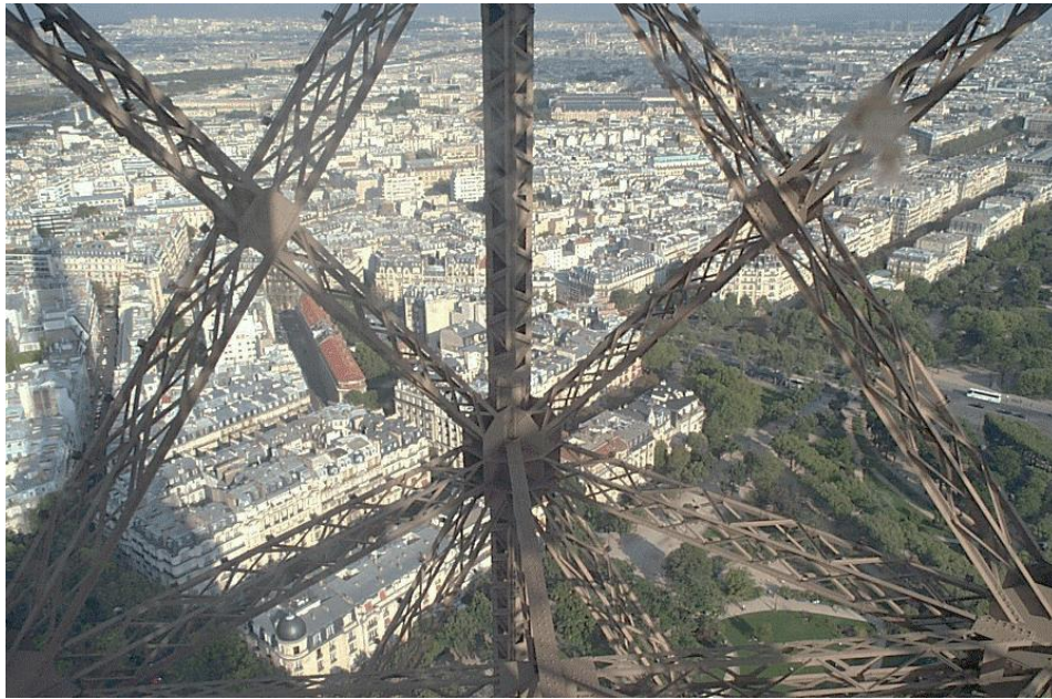
Figure 15.2 – Truss structure of the Eiffel Tower
