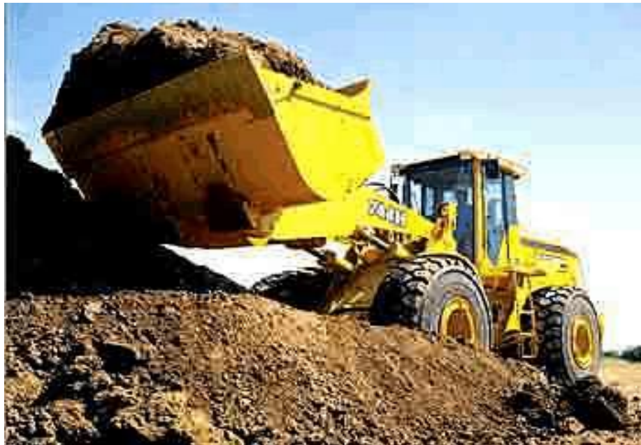
Figure 8.5 – Loader collects crushed stones
