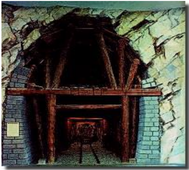
Figure 9.5 – Construction of Mont Cenis Tunnel
