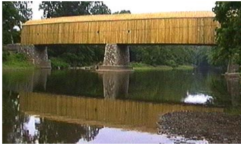
Figure 1.1 – Old covered bridge
