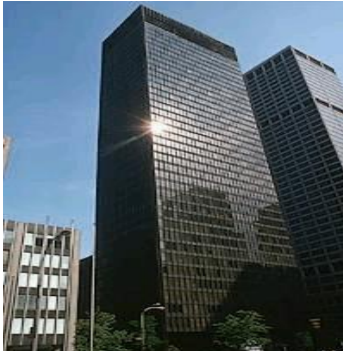
Figure 5.1 – The curtain wall of Mies van der Rohe’s Seagram Building, New York City
