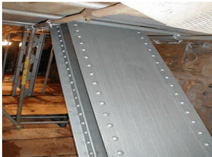
Figure 5.2 – Riveted structure
