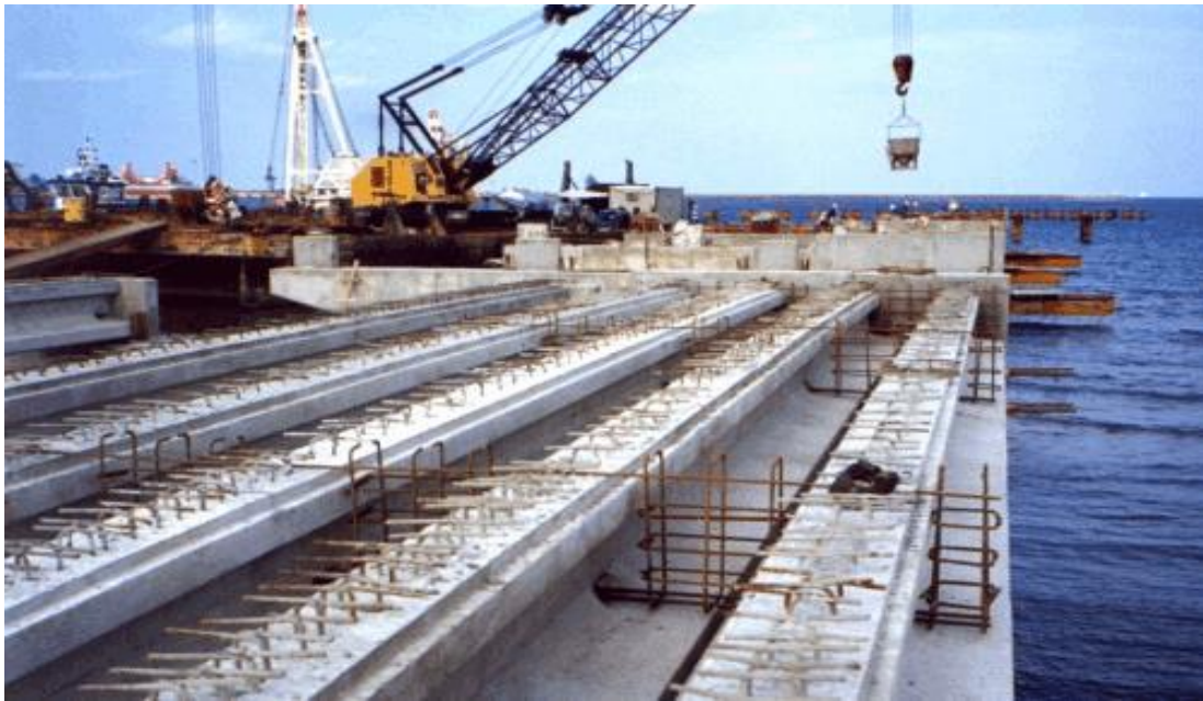
Figure 5.4 – Prestressed beams launched and reinforcement diaphragm tied
