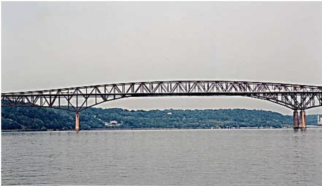
Figure 10.3 – Newburgh-Beacon Bridge, New York
