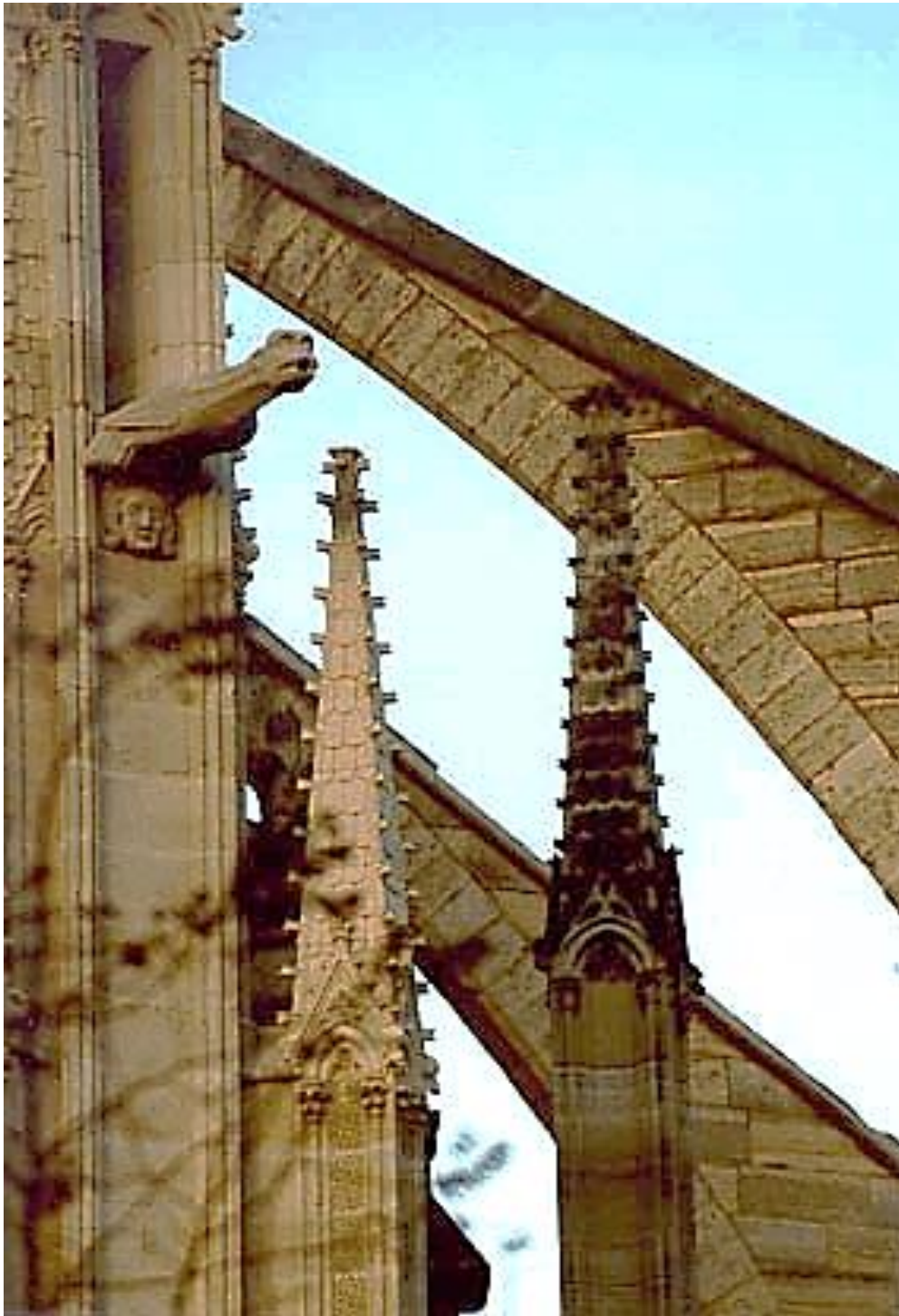
Figure 14.2 – Flying buttress
