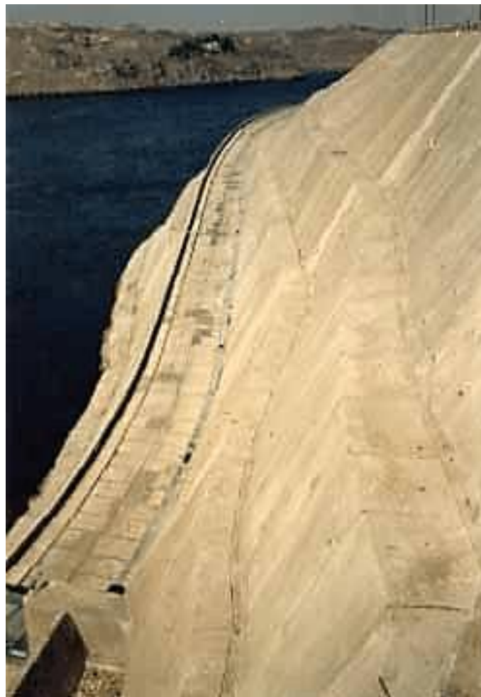
Figure 4.1 – Aswan High Dam, Egypt
