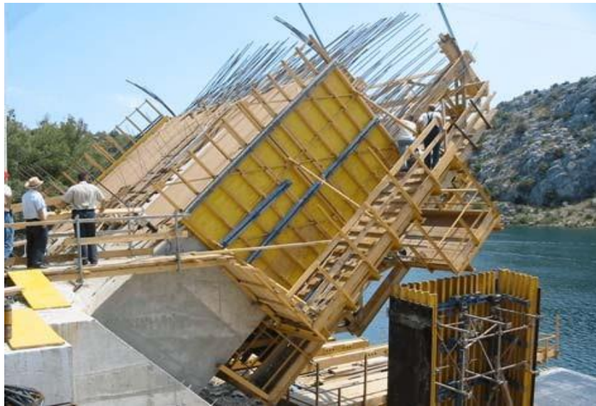
Figure 4.2 – The shuttering
