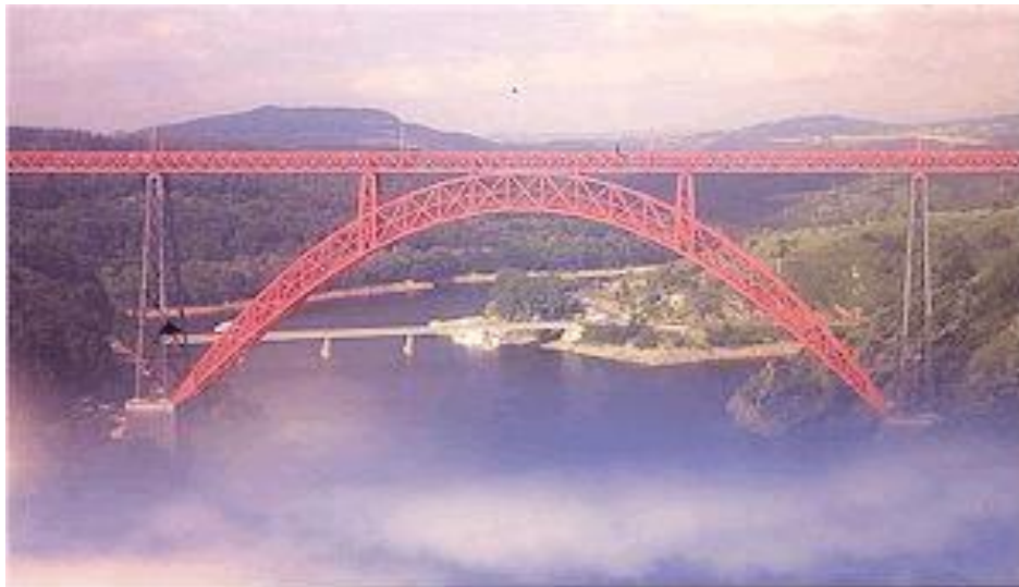
Figure 15.3 – Garabit Viaduct, France
