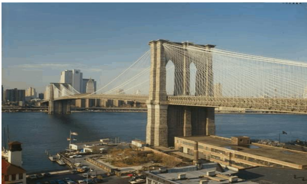
Figure 10.4 – Brooklyn Bridge, New York
