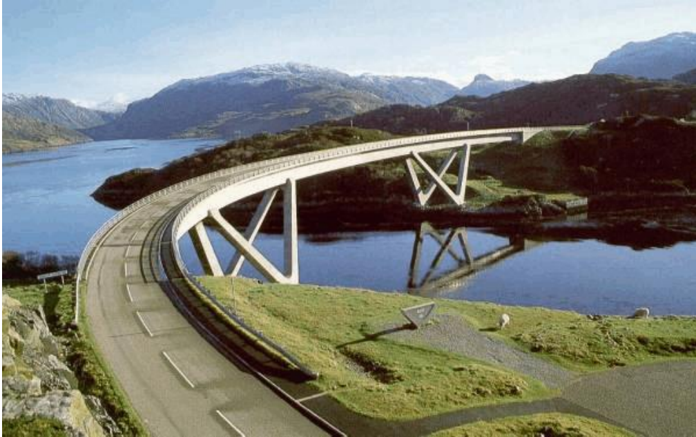
Figure 5.6 – Kylesku prestressed concrete bridge, Scotland
