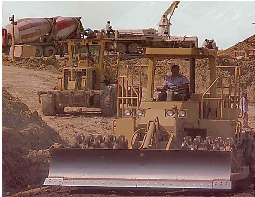
Figure 8.3 – Bulldozer pushes and spreads earth
