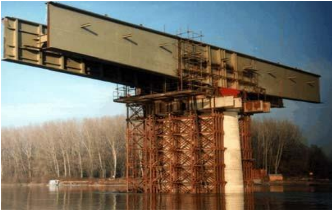
Figure 11.3 – Cantilevering of a bridge
