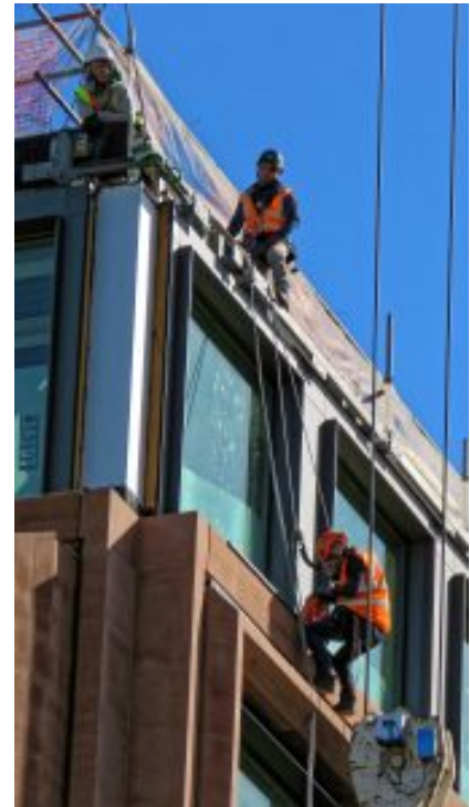
"Construction workers" by Acabashi , CC BY-SA 4.0
