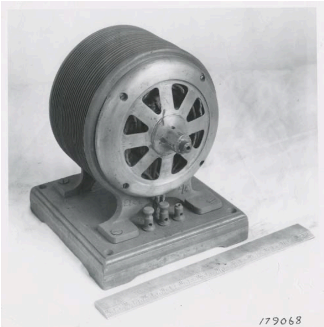
Figure 2. Tesla's polyphase motor, 1888. University of Pittsburg Library System, Historic Pittsburg, George Westinghouse Museum Collection, 20170323-hpichswp-0044, https://historicpittsburgh.org/islandora/object/pitt%3A20170323-hpichswp-0044 (accessed August 15, 2019). Public domain.
