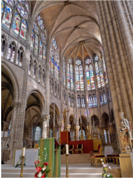
The chancel at the basilica of Saint-Denis in France that illustrates both the cross-ribbed vaulting and pointed arches characteristic of Gothic churches.
