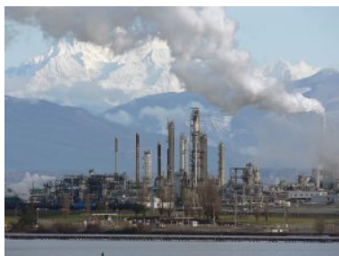
Anacortes, Washington Refinery
