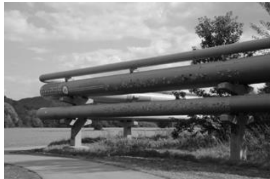
Figure 4.18 Above ground district heating pipes in Jena (Public Services Energie Jena-Pössneck).
