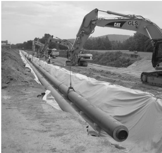
Figure 4.19 District heating pipes will be lifted into the trench [51].
