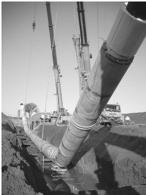
Figure 4.21A prefabricated culvert is lifted into the culvert channel placed into the riverbed on rolls [51].
