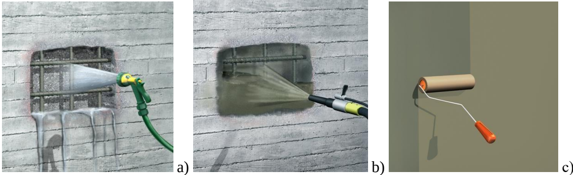
Fig. 3. Mechanized repair concrete.
