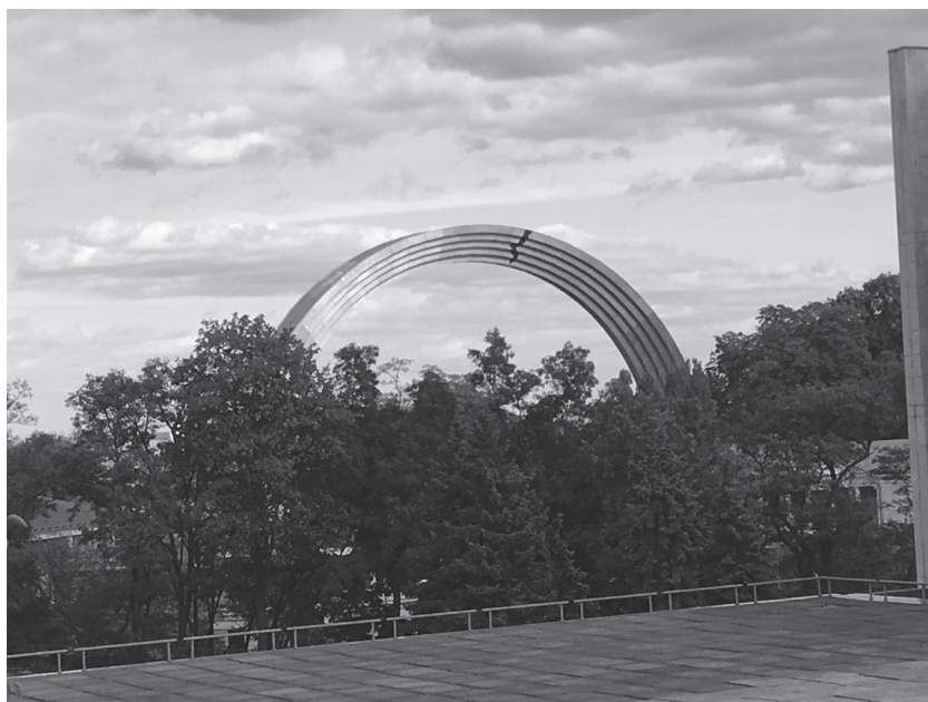
Figure 4.4 Cracks in the friendship: People's Friendship Arch in Cross Park, Kyiv, 1 October 2019. Photo by authors
