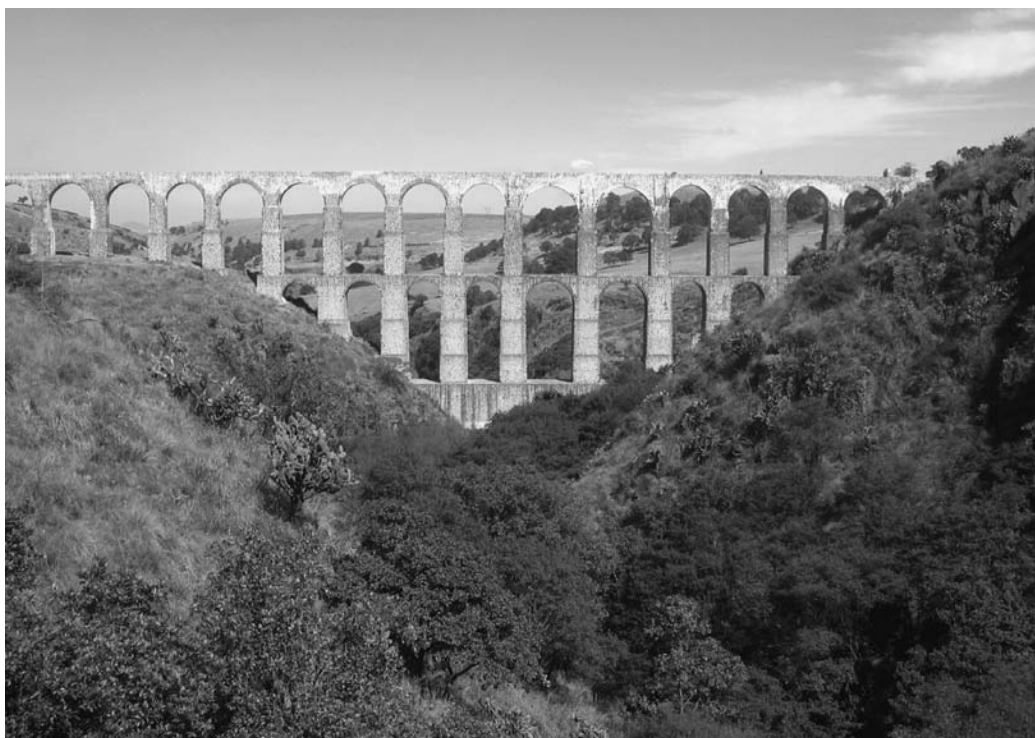
Figure 4.1 Xalpa aqueduct, about 15 km northwest of Tepotzotlán, built in the 1700s
