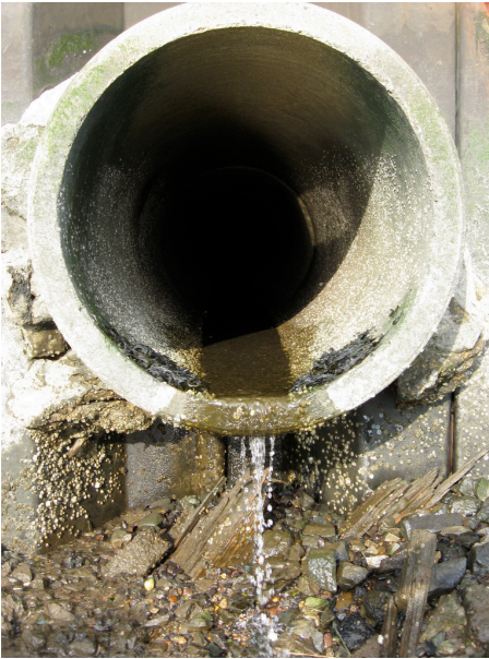
A likely combined sewer overflow outlet in Bayonne, NJ.
