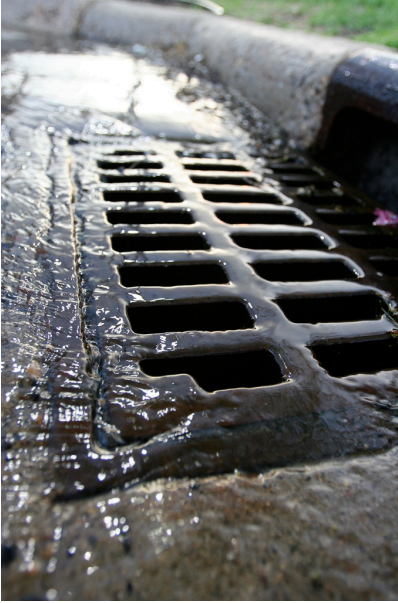
Melted water flows down through the manhole
