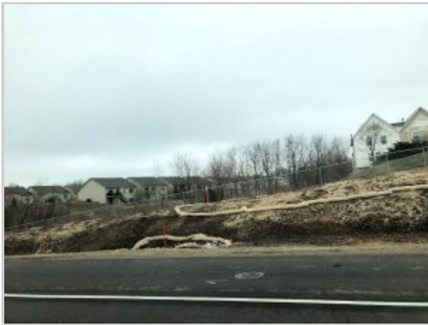
New construction is particularly sensitive to erosion, this disturbed shoulder off of I-35 near Ankeny is using a few techniques to control erosion-straw waddles and straw to help grass seed establishment. Photo Credit: Amber Anderson.
