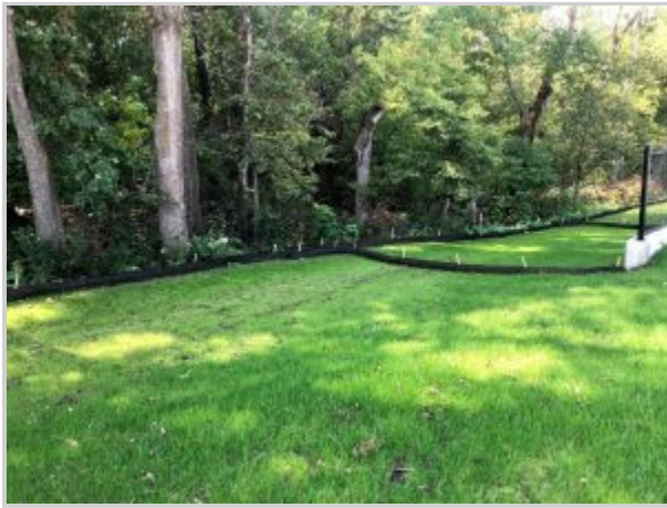
As the perennial cover of grass gets established next to the new Ames High School, these black strips are used to slow water and stop sediment moving down the hill. Photo credit: Amber Anderson.
