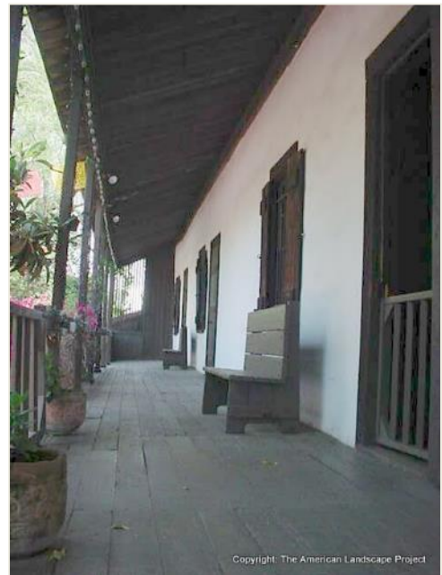
Figure 2-29: Los Angeles, CA - The Avila Adobe is reputed to be the oldest house in Los Angeles. It is remarkably cool inside, even on very hot days. It is a museum now on Olvera Street, a tourist district near downtown.
