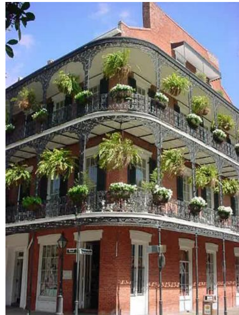
Figure 2-27: New Orleans, LA. – The beautiful wrought-iron gallery porches on this building in the French Quarter were popularized during the period when Spain ruled Louisiana. Note the effective shade the porches provide to the building’s walls.
