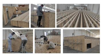
Figure 1. Construction of test floor.
