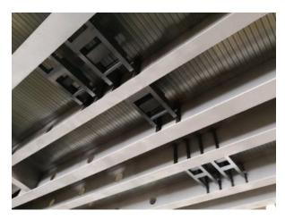
Figure 17. TMDs installed on-site.
