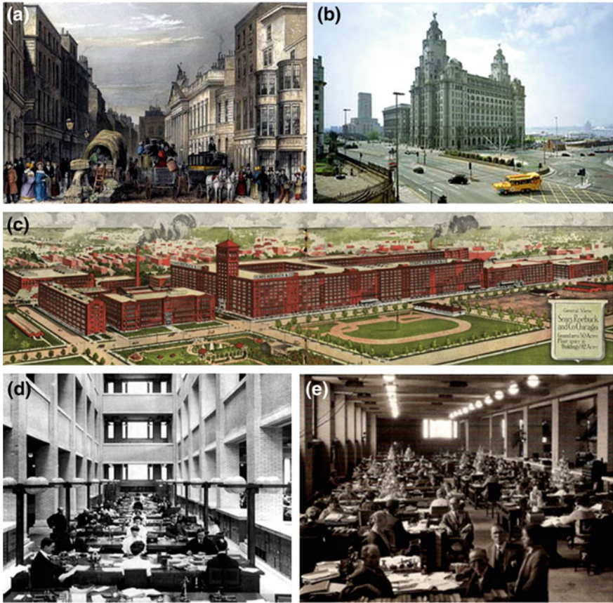
Fig. 1.2 a East India Co., Leaden Hall Street, London (1729; 1726); b Oriel Chambers, Liverpool, UK (1864); c Sears, Roebuck and Co., Chicago, USA (1905–6); d, e Larkin Building, Buffalo, NY (1904)
