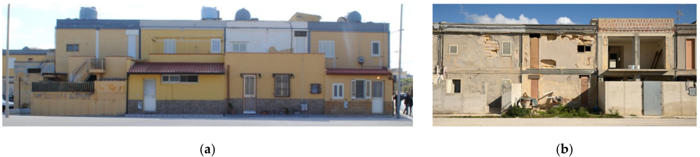
Figure 2. Unauthorized additions in the Cappuccinelli district: private gardens occupied by new rooms (a) and other chaotic modifications (b) in the terraced block named “L”.
