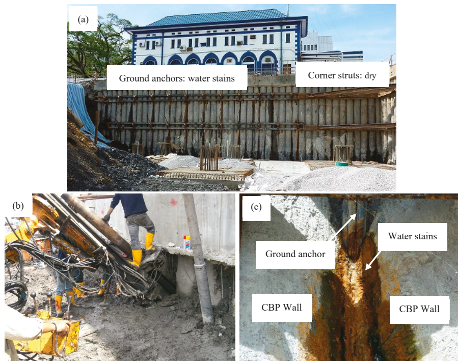
Figure 7. (a) Groundwater leakage from where ground anchors were installed; (b) drilling of ground anchor in between bored piles; and (c) close-up of the water leakage from the ground anchor.
